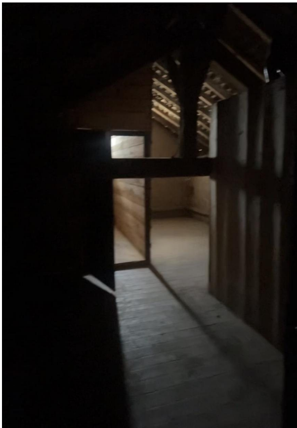
Attic today — dark; daylight is a prerequisite for habitable use.
