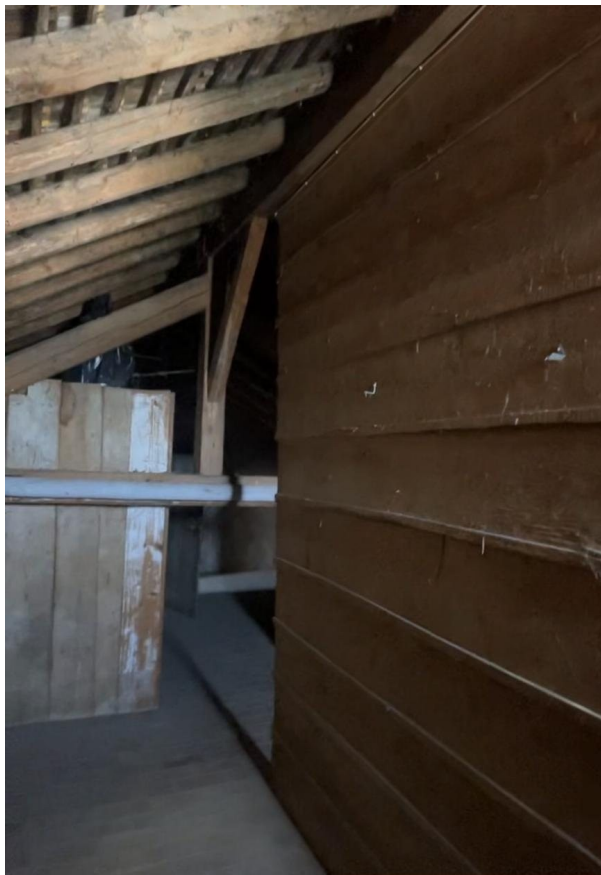
Charpente dry and sound; struts bear on the outer walls.
